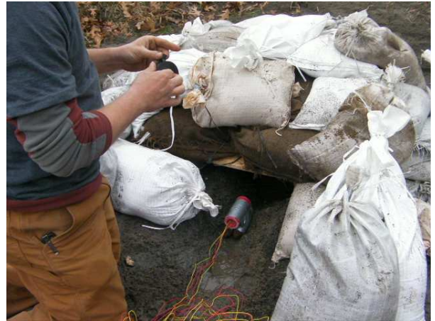
Preparing the bunker
